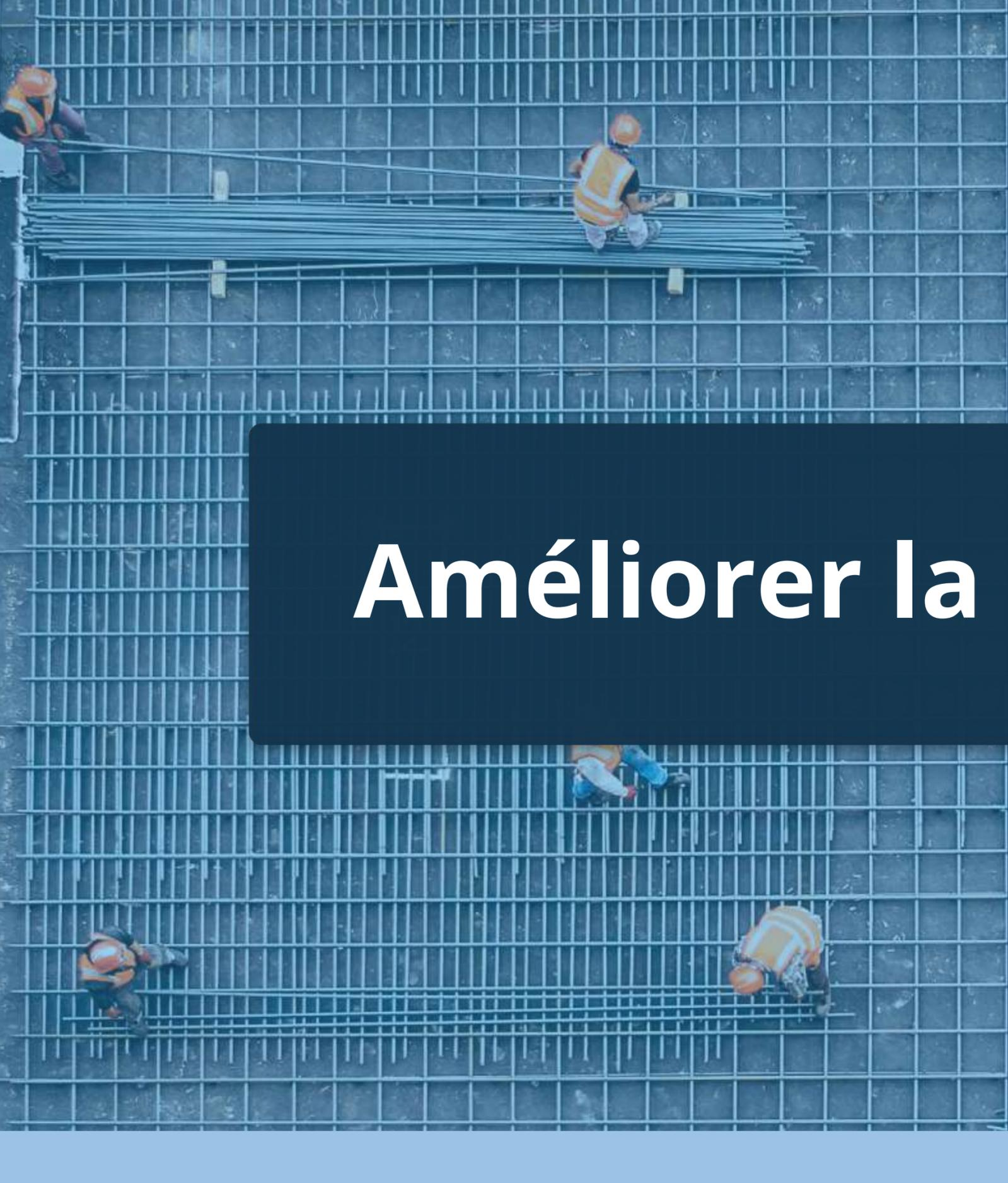
An aerial photograph of a construction site showing a grid of steel reinforcement bars (rebar) laid out on a concrete surface. Several workers wearing orange safety vests and hard hats are visible, working on the grid. A large black rectangular box is overlaid on the center of the image, containing the text 'Améliorer la collaboration'.
